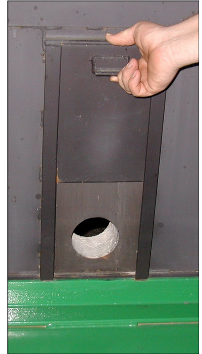
Access Door for Lighting
