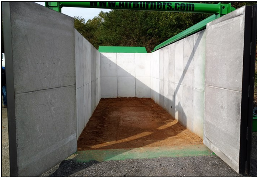
S327 FireBox Rear Doors (Open)
