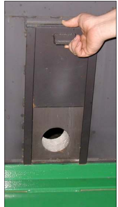
Access Door for Lighting
