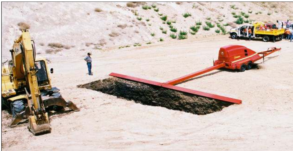
Trench Burner Positioned at a Perfect Pit
