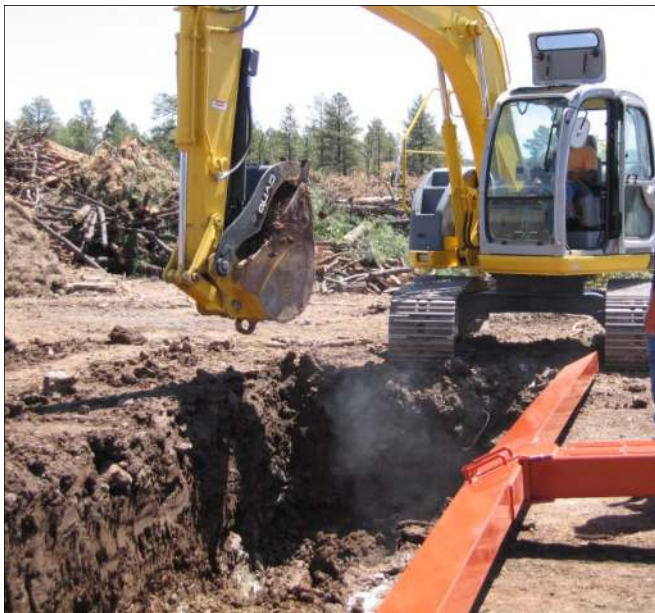
Pit Excavation with Manifold Positioned
