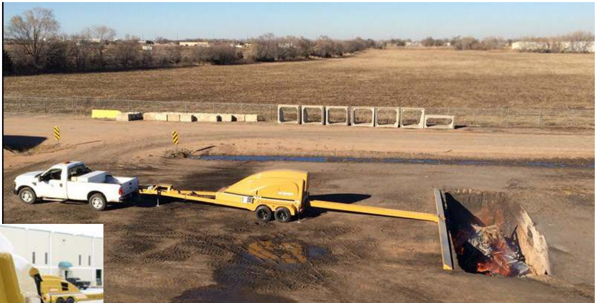
T300 Positioned at Trench
