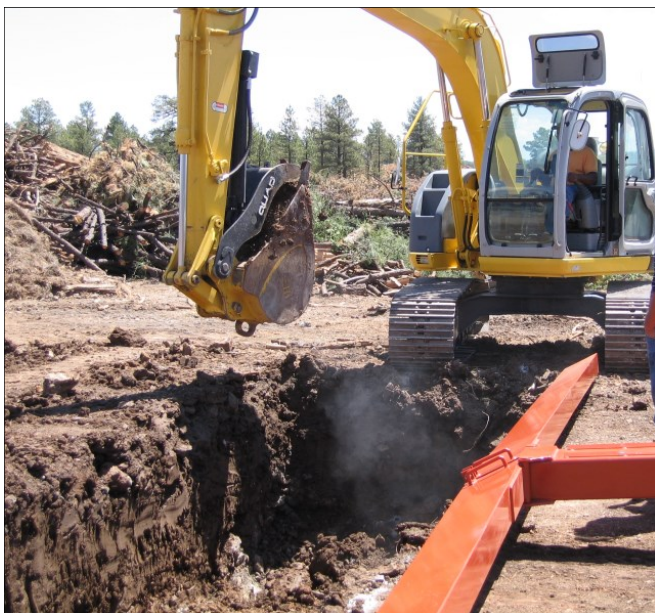
Pit Excavation with Manifold Positioned
