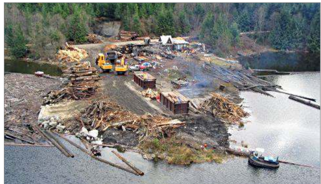
Hydro Dam Reservoir Waterborne Debris Elimination by multiple S327 Air Curtain Burners
