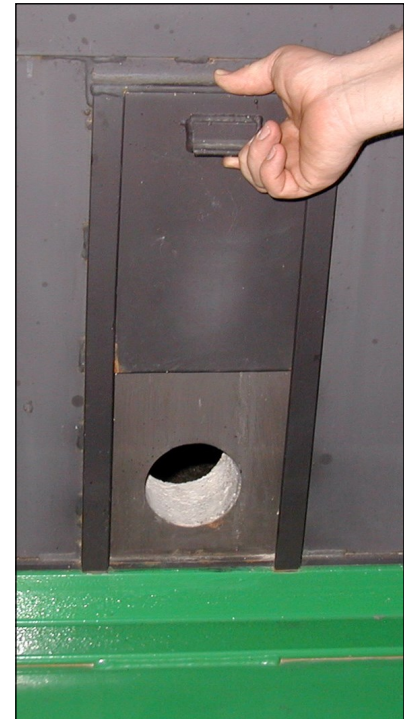
Access Door for Lighting
