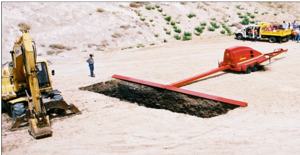
Trench Burner Positioned at a Perfect Pit
