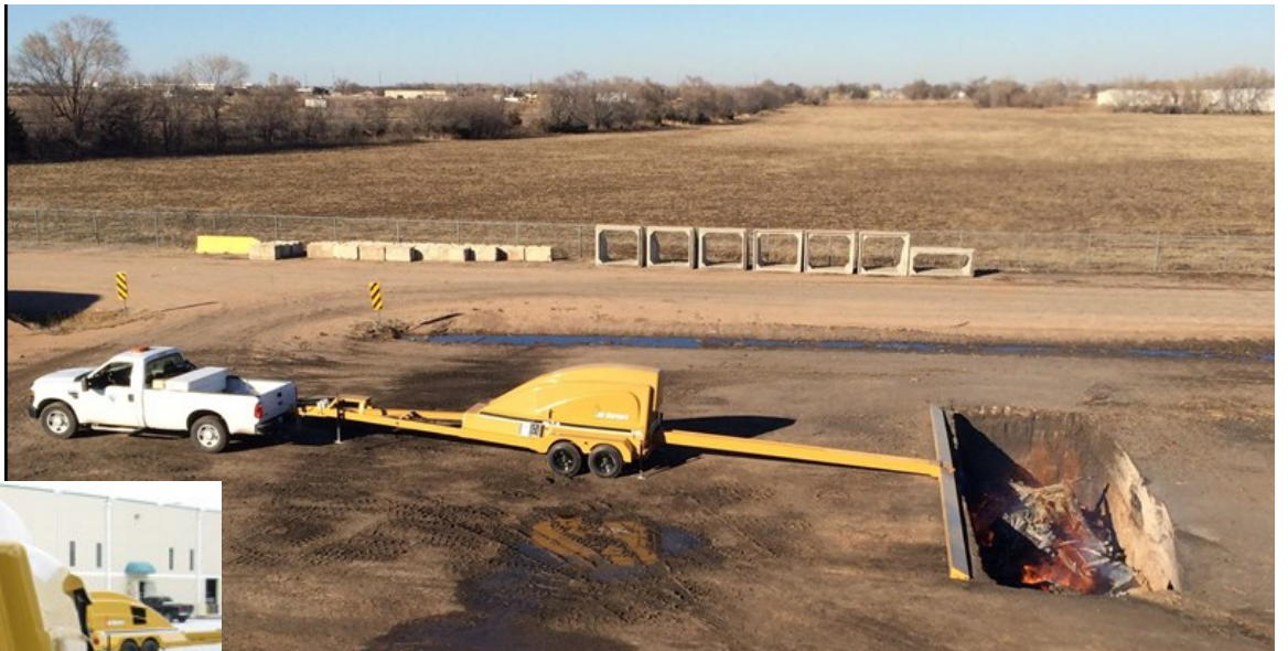
T300 Positioned at Trench
