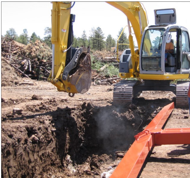
Pit Excavation with Manifold Positioned
