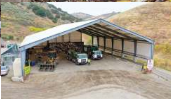
Above: Fabric-clad Truss Arch frames allow for natural lighting with the option of supplemental electric lighting. Left: Steel I-beam frames can be customized for optimal ventilation, easy maneuvering and waste transfer.
