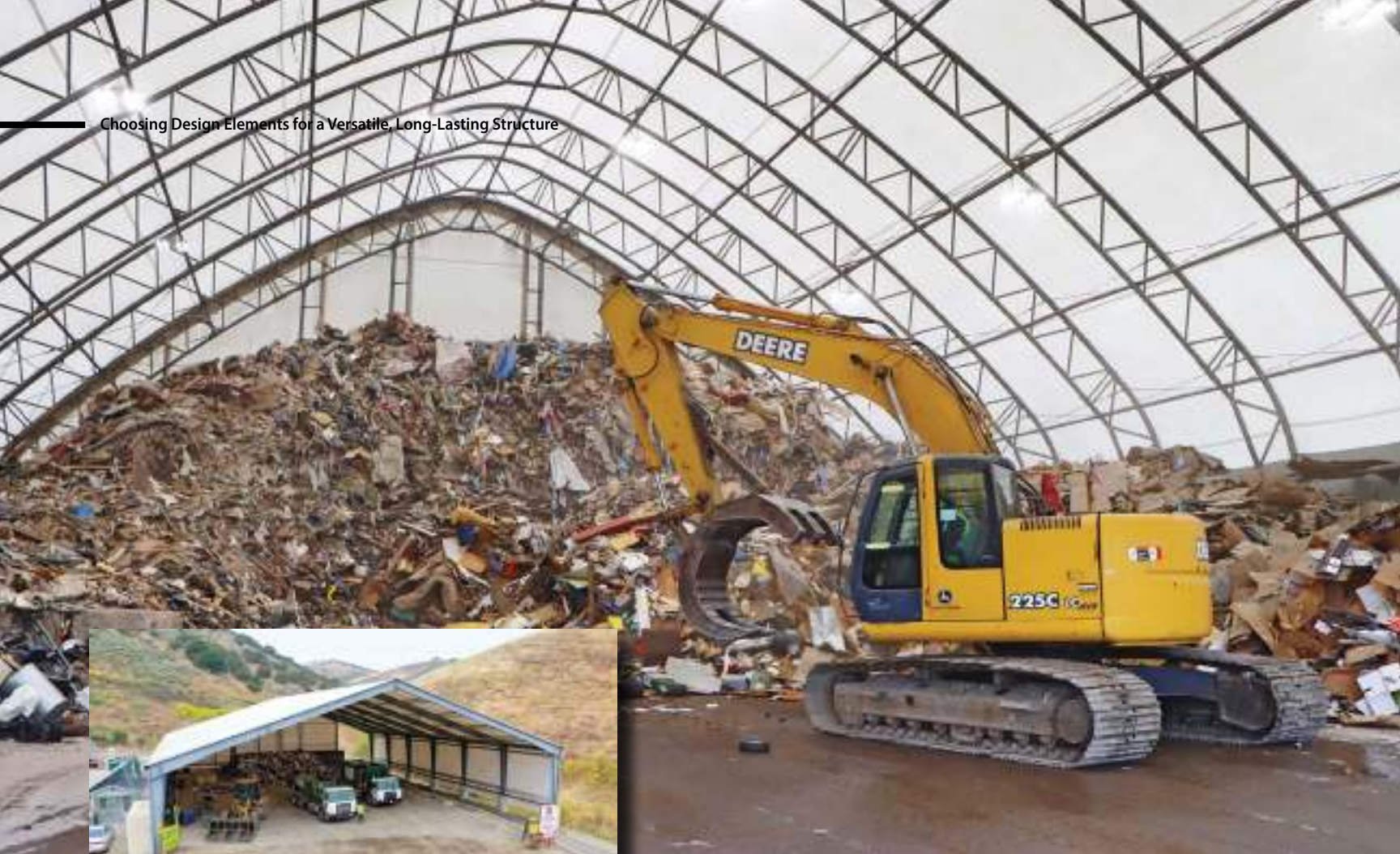
Above: Fabric-clad Truss Arch frames allow for natural lighting with the option of supplemental electric lighting. Left: Steel I-beam frames can be customized for optimal ventilation, easy maneuvering and waste transfer.
