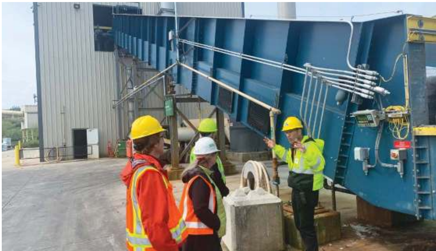
After visual inspection for non-conforming items, waste is sent to a rough shredder, baled, and fed into the Juno™ Clave via conveyor belt.
